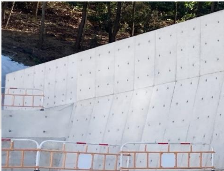
External Surface of U-trough
